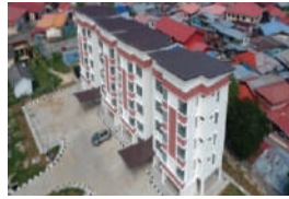
Hospital Semporna Quarters, Sabah
