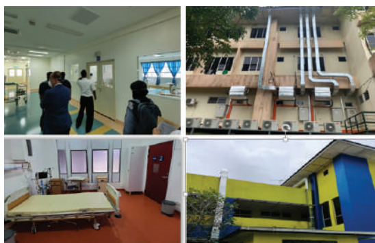
Image 6.12 Isolation Room Upgrading Works
